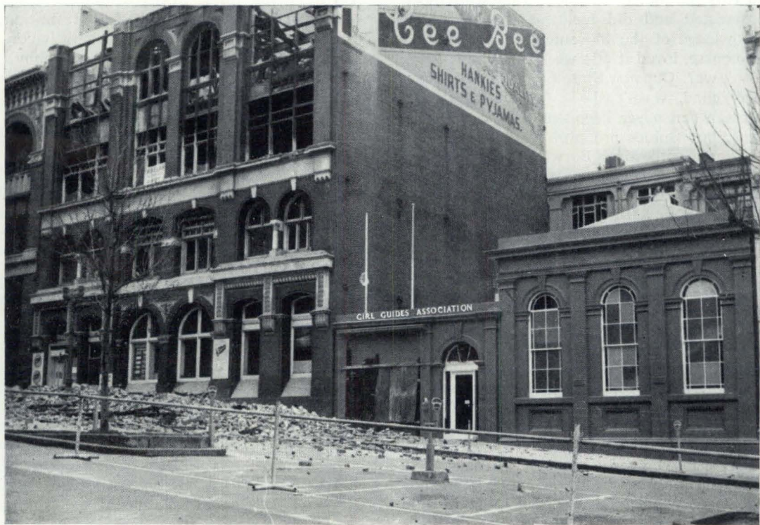
Headquarters after the Brooks Building fire, 2nd July, 1962.
